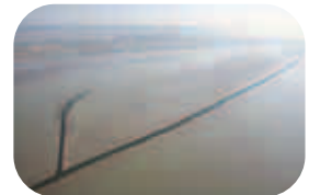
Supporting operations for Port 2000: building a breakwater to promote the formation of a mud bank
