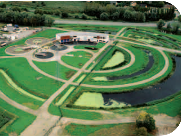
Aerial view of a Filtration Garden
