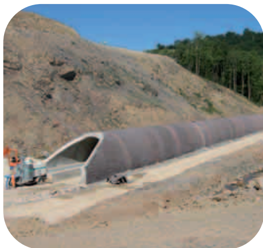
Construction is integrated into the landscape
