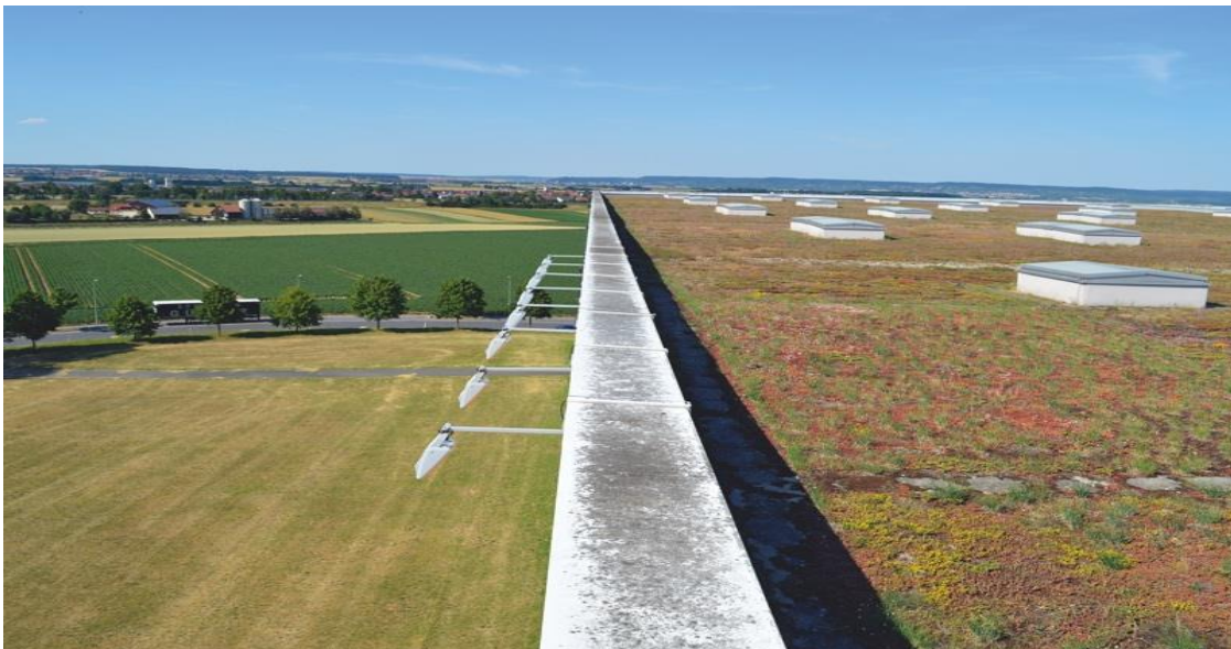
Figure 13. An example of green roof on a large industrial building.
